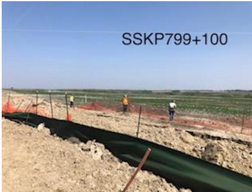
Removing damaged snow fence
