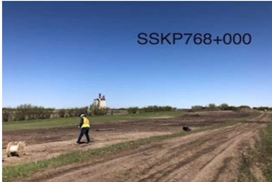
Pipe yard – raking up smaller pieces in piles
