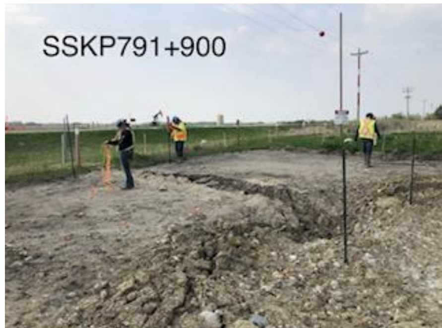
Roping off an area where the soil settled over mainline
