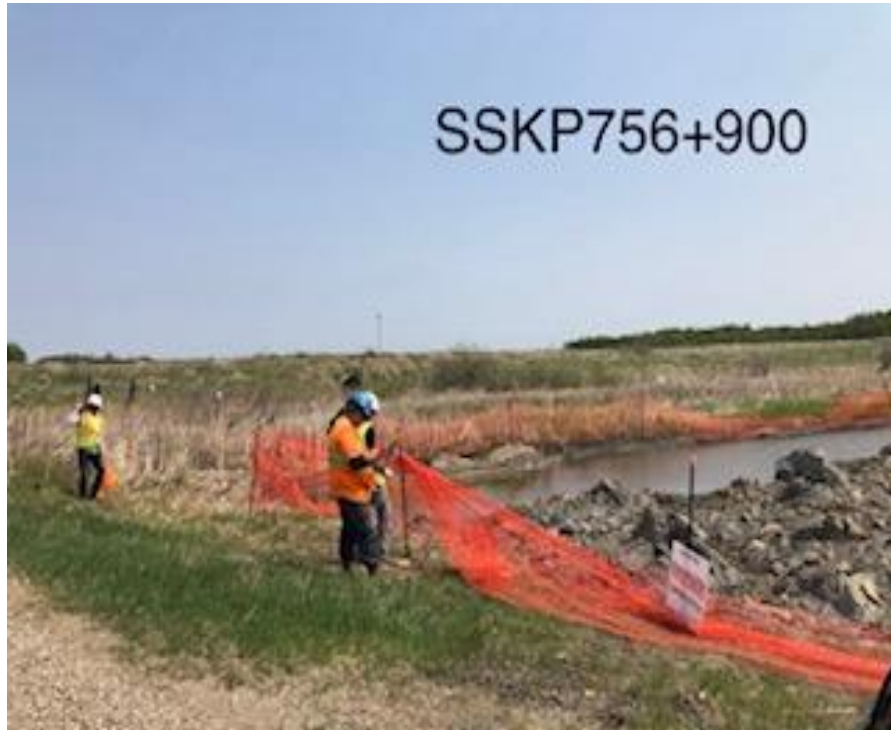
Repairing snow fence around wet land area
