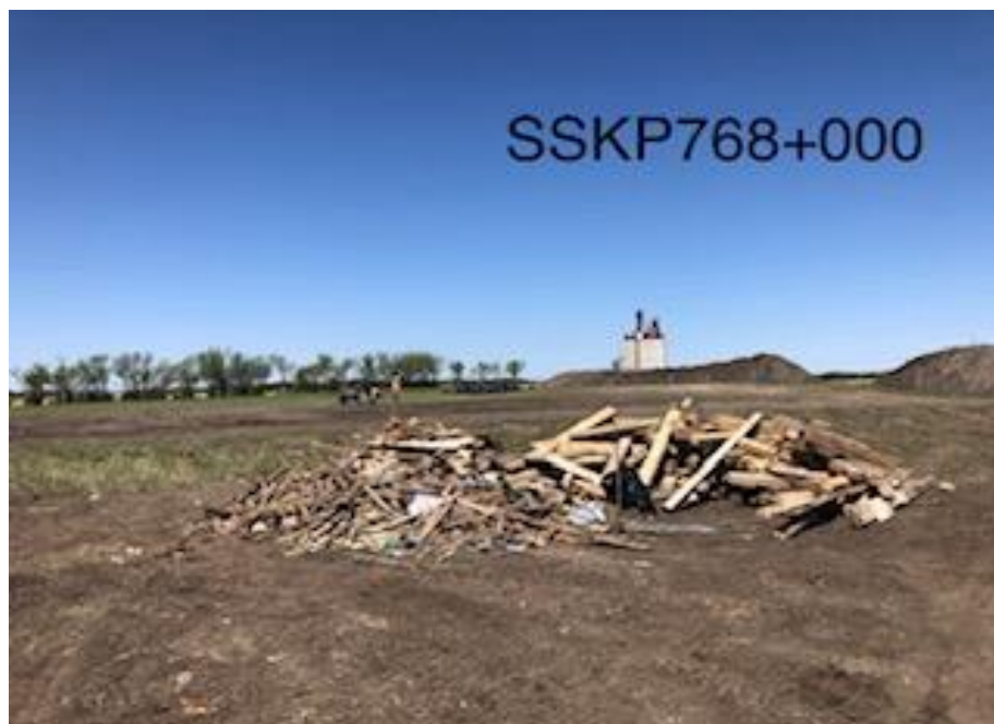
Debris pile – skids
